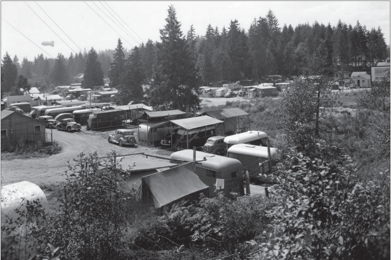
War-time workers lived in trailers, shacks, even chicken coops, as they poured into Bremerton in 1942. Note the barrage balloon on the horizon. The balloons were tethered to the ground by steel cables that could slice the wings off low-flying enemy aircraft. Puget Sound Navy Museum
