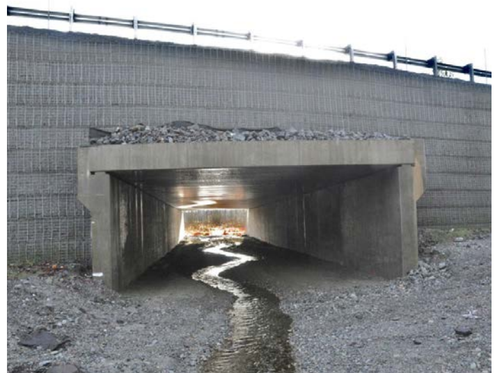
Figure 13. The new crossing is 24 foot (7.32 m) wide by 12 foot (3.66 m) tall and provides 0.97 miles (1.57 km) of upstream habitat for coho, steelhead, and resident trout. The large opening will also allow small and medium sized animals such as deer to cross safely under the highway.
