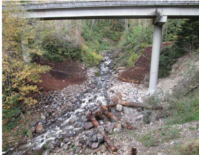
Figure 17. The debris were removed under the bridge during a seismic retrofit project now allowing access for Chinook, coho, and pink salmon, steelhead, and resident trout to 16.71 miles (26.89 km) of upstream habitat.
