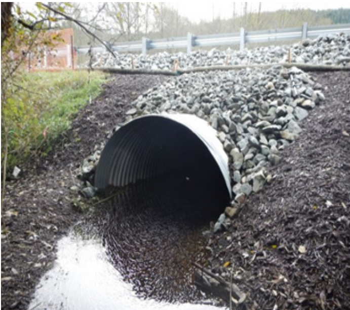
Figure 28. This new 8 foot (2.44 m) round, corrugated steel culvert replaced an undersized 1.5 foot (0.46 m) culvert. This project provides upstream habitat for coho, steelhead, searun cutthroat and resident trout.
