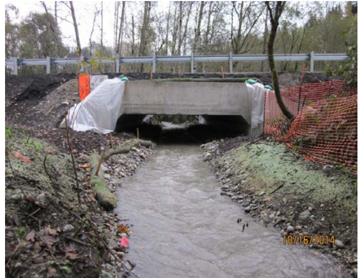
Figure 21. The new crossing is a 19 foot (5.8 m) box culvert that provides upstream habitat for coho, steelhead, searun cutthroat and resident trout.
