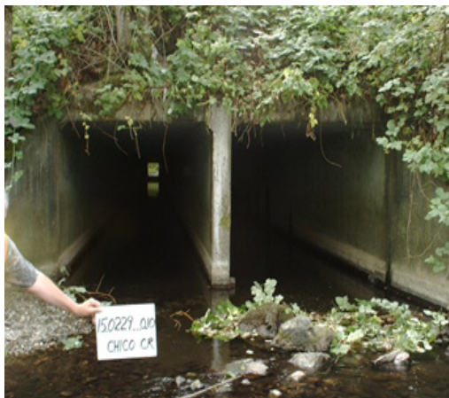
Figure 5. The SR 3 culvert before the log control and baffles were installed.
