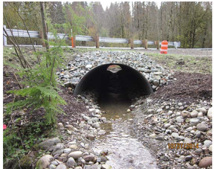
Figure 19. The new crossing is a 9 foot (2.74 m) culvert that provides upstream habitat for coho, steelhead and resident trout.
