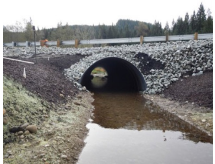
Figure 27. The new structure is a 10 foot (3.05 m) round, corrugated steel culvert, providing upstream habitat for coho, steelhead, searun cutthroat and resident trout.
