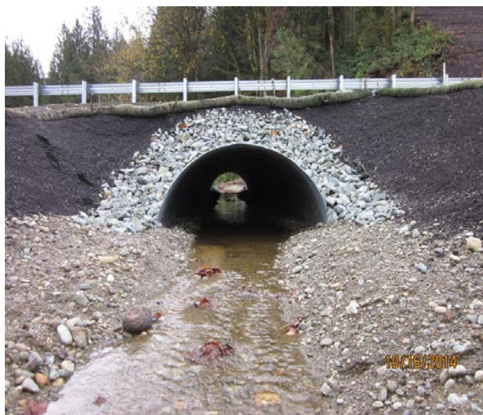
Figure 23. The new crossing is a 9 foot (2.74 m) culvert that provides upstream habitat for coho, steelhead, searun cutthroat and resident trout.
