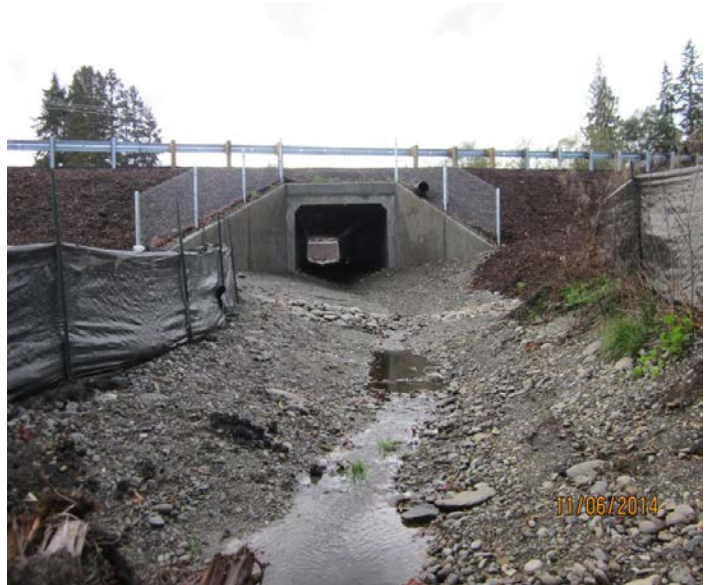
Figure 15. The new crossing is a box culvert 10 foot (3.05 m wide) by 10.5 foot (3.2 m) tall. This structure will provide fish passage and wildlife passage for small and medium sized wildlife such as raccoon and deer.
