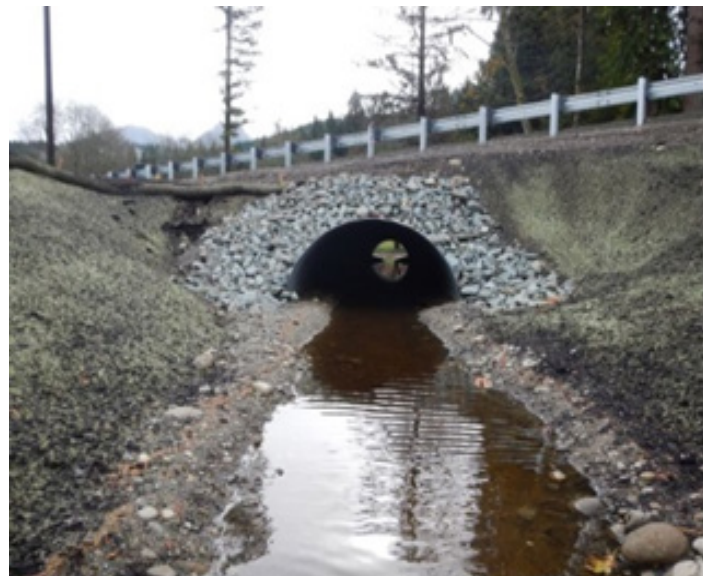
Figure 25. The new structure is an 8 foot (2.44 m) round, corrugated steel culvert, providing upstream habitat for coho, steelhead, searun cutthroat and resident trout.
