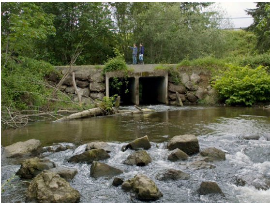
Figure 4. Kittyhawk Drive (Kitsap County) culvert just downstream of the SR 3 culvert.
