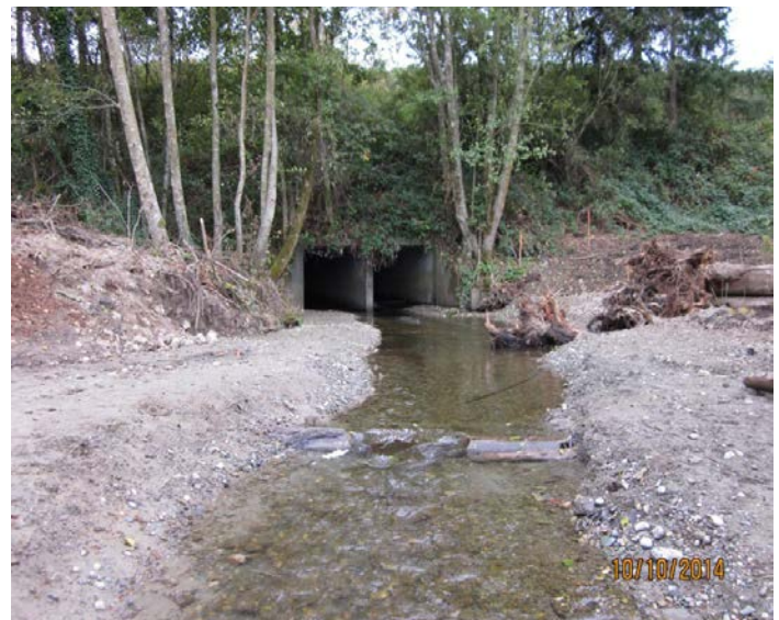
Figure 6. The SR 3 culvert after removal of the Kittyhawk Drive culvert that was just downstream of it. This will open up 21.77 miles (35.04 km) of upstream habitat for chum, Chinook, and coho salmon, steelhead, searun cutthroat and resident trout.
