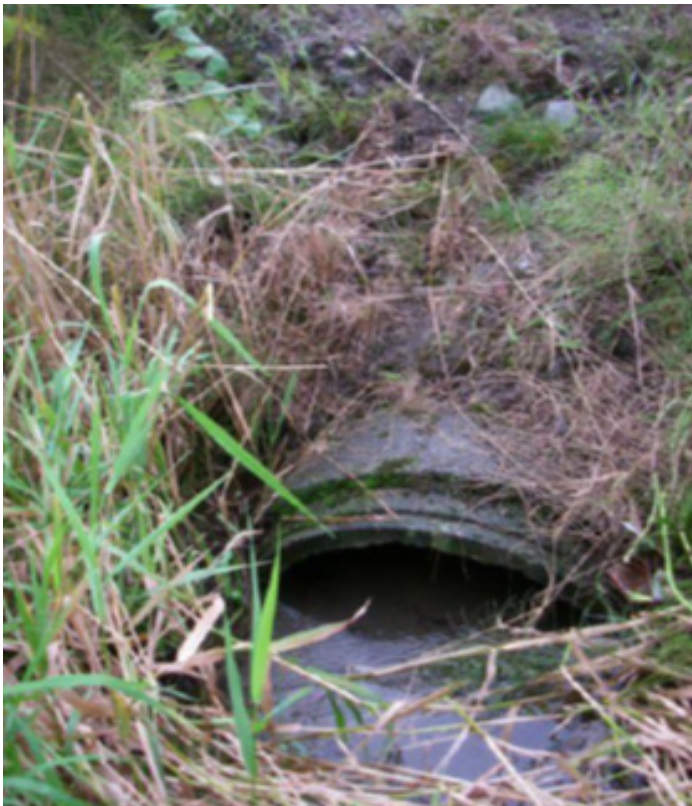
Figure 26. The old crossing was a 3 foot (0.91 m) round, concrete culvert. While this culvert was considered passable for fish, it was undersized for the watershed.
