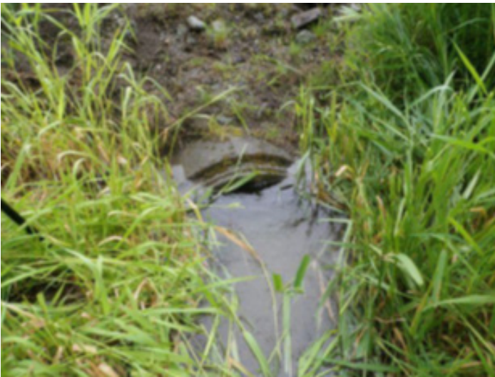
Figure 24. The old crossing was a 3 foot (0.91 m) round, concrete culvert. While this culvert was considered passable for fish, it was clearly undersized for the watershed.
