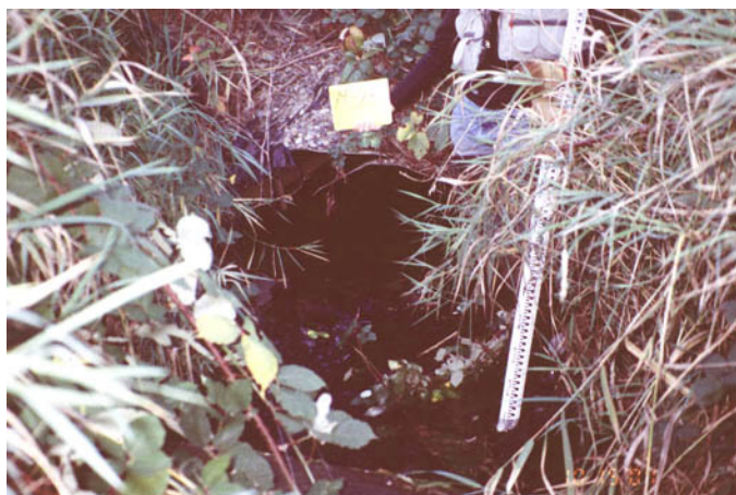
Figure 9. The old crossing consisted of twin 3.5 foot (1.07 m) round culverts that were velocity barriers.
