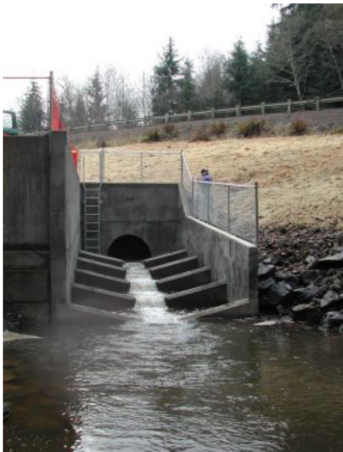
Figure 31. An example of a durable and efficient fishway on SR 401 at milepost 8.8 for Cement Creek.
