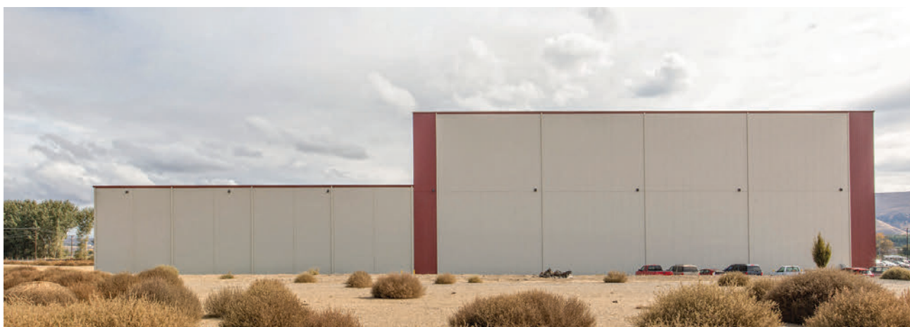
The exterior of the Matson Fruit cold storage warehouse in Selah, Washington. The right side of the warehouse, with steel siding and insulation, was built to allow higher stacking of pallets using robotic cranes. The left side of the warehouse, with concrete siding, is similar in size to a standard cold storage facility.
