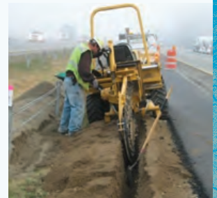
Digging a trench for fiber in a right of way. Source: WSDOT
