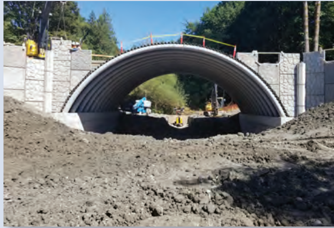
Building up around the SR 203 Loutsis Creek arch culvert
