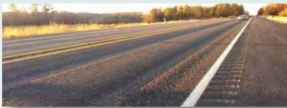
Ruts from studded tires damage roads throughout the state.
