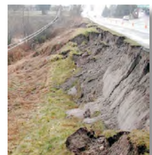
Martin Way Landslide Damage.
