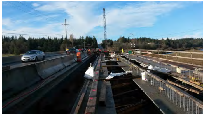
Travelers use the completed southern half of the Davis Slough Bridge while WSDOT crews work to complete the northern half in December 2015.
