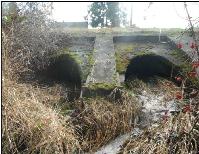
Figure 6. The old crossing was a two-cell concrete culvert of with each cell measuring 5.3 ft span by 3.7 ft rise that was a barrier to fish passage due to slope.
