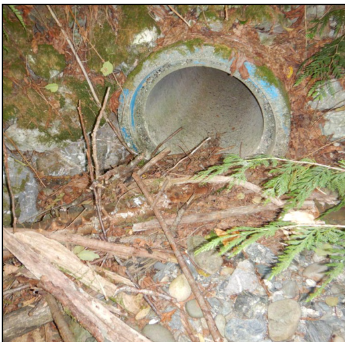
Figure 8. The old crossing was a 2.5 ft diameter culvert that was a barrier due to excessive slope and hydraulic drop at the outlet.
