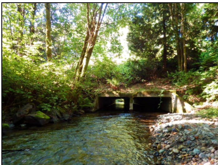
Figure 20. The old crossing was a two-cell box culvert with each cell measuring 8 ft span by 6 ft rise. The culvert was a barrier due to velocity and accumulated debris.
