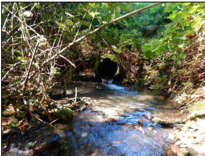
Figure 12. The old crossing was a 103 ft long, 2ft diameter concrete culvert that was a barrier due to slope.
