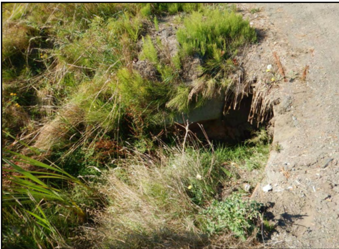
Figure 22. The old crossing was a 3 ft diameter culvert that discharged mid-length into the Bagley Creek culvert and was a barrier due to hydraulic drop.
