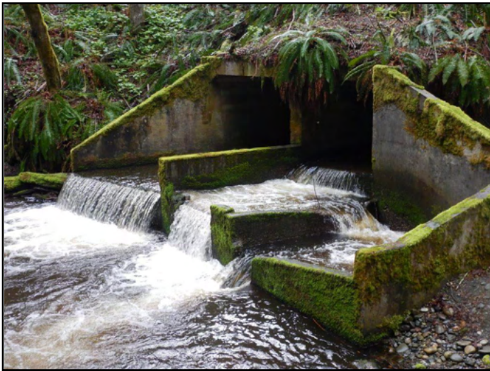
Figure 26. The old crossing was a 7 ft span by 7 ft rise double cell box culvert that was retrofitted with a concrete weir pool fishway on one cell to facilitate fish passage. The fishway was assessed as a barrier due to low depth of flow and high velocity.
