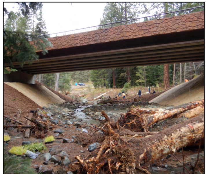
Figure 31. The new crossing is a 100 ft span bridge that restores connectivity to approximately 3.4 miles of spawning and rearing habitat for steelhead, resident rainbow trout, and bull trout. The Swauk Creek Projects received the 2021 Environmental Excellence Director's Award for commitment to collaborative partnerships, tenacity, and dedication to environmental excellence.
