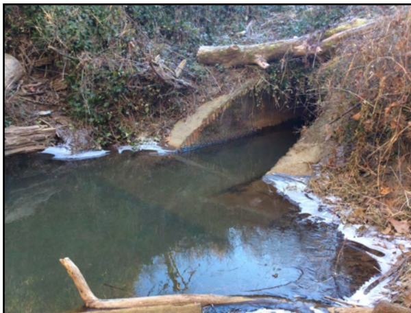
Figure 28. The old crossings were a 6.75 ft round structural plate steel culvert and an 8.25 ft round structural plate steel culvert.
