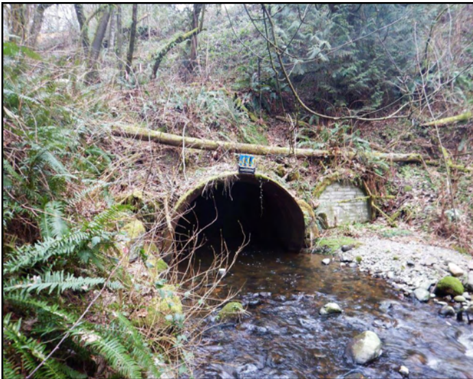
Figure 18. The old crossing was a 216 ft long by 10.8 ft diameter smooth steel culvert retrofitted with interior baffles that was a barrier due to excessive velocity and hydraulic drop over the baffles.
