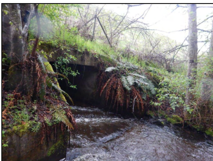
Figure 24. The old crossing was a 5 ft span by 5 ft rise by 332 ft long concrete box culvert retrofitted with 62 steel baffles inside and two bed controls downstream to facilitate fish passage on mainstem Bagley Creek. The fishway was determined to be a barrier due to excessive hydraulic drops over the bed controls. The long culvert also conveyed Bagley Creek under James Page Road.
