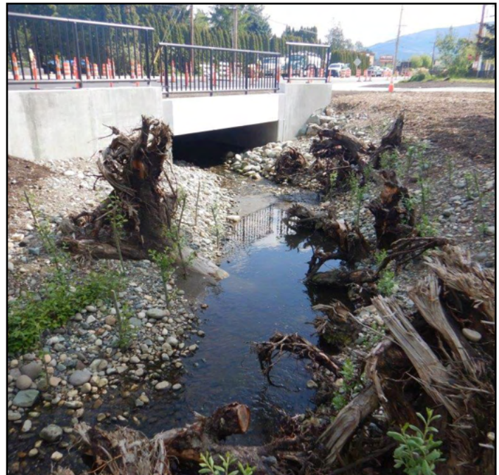
Figure 7. The new crossing is a 15.6 ft span by 8.5 ft rise concrete culvert. Adult salmon were observed in the creek shortly after rewatering the stream.
