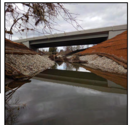
Figure 29. The new crossings are a 22 ft span by 15.3 ft rise concrete culvert that is 71.2 ft in length and a 125 ft span bridge. A bridge was selected for the more downstream structure due to the backwatering effect of the Chehalis River. Both structures experienced a 100-year flood event shortly after construction.
