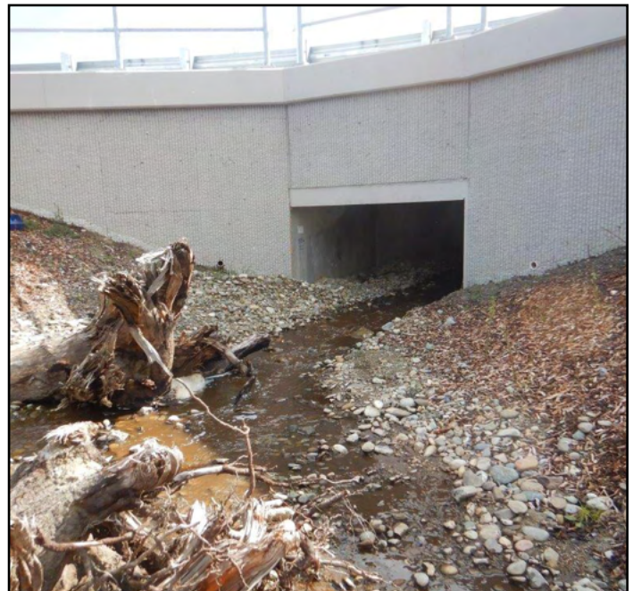
Figure 23. The new crossing on the tributary is an 8 ft span by 8 ft rise concrete box culvert. The unnamed tributary was realigned so that open channel could be created between S. Bagley Creek Road and James Page Road.
