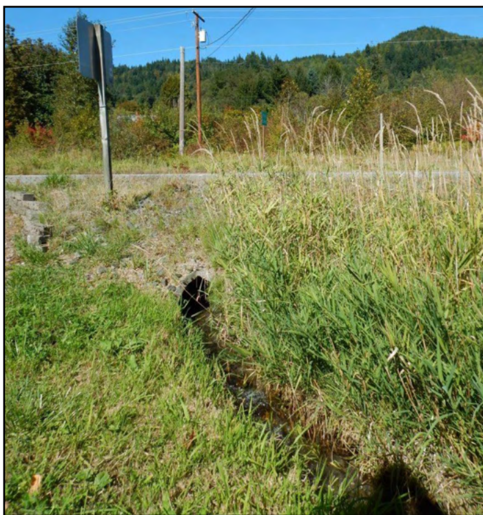
Figure 10. The old crossing was a 77 ft long, 2 ft diameter concrete culvert that was assessed as a barrier due to excessive velocity.
