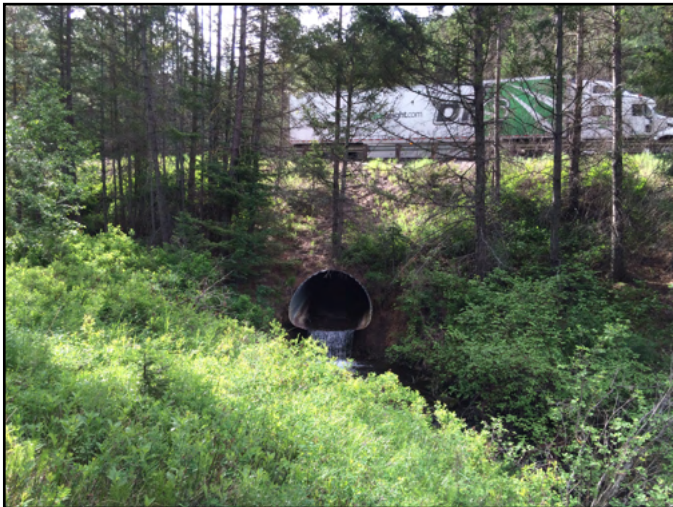
Figure 30. The old crossing was a 6 ft span by 9 ft rise by 118 ft long multi-plate steel culvert that was a barrier due to a hydraulic drop at the outlet.
