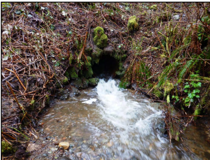
Figure 14. The old crossing was a failing 2 ft diameter corrugated metal culvert that was 102 ft long. This project benefits steelhead, coastal and resident cutthroat trout.
