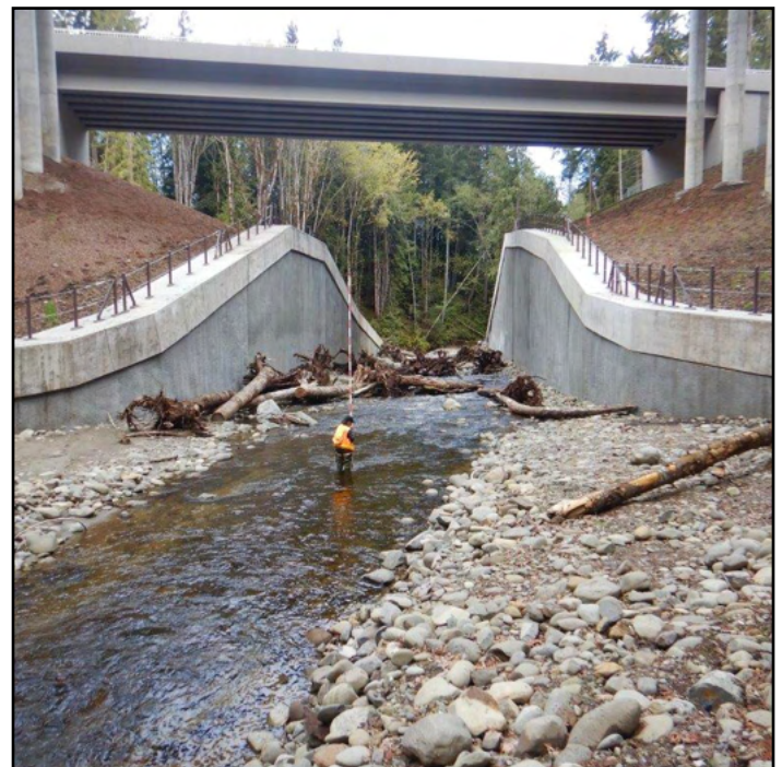
Figure 27. The new crossing is a full span bridge with secant pile walls to stabilize the bank slopes, as this area is geologically prone to landslides. The span between the walls is 50 ft. Adult Chinook salmon were observed within the project area and upstream of the new bridge during the Post-Construction Monitoring Inspection, which is the first documented observation of chinook utilizing Siebert Creek.
