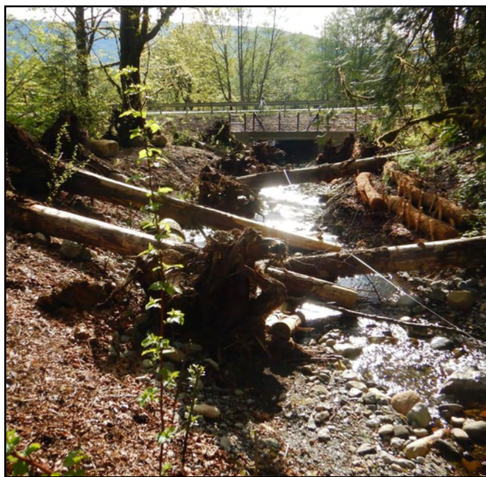
Figure 9. The new crossing is a 14.3 ft span by 10 ft rise concrete culvert. Also in 2021, the private landowner of the next downstream crossing replaced a barrier culvert with a bridge.
