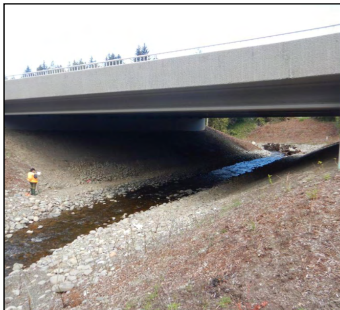
Figure 25. The new crossing on Bagley Creek is a 126 ft span bridge. This project also includes two new county owned fish passable structures under James Page Road – one for mainstem Bagley Creek and one for the unnamed tributary.
