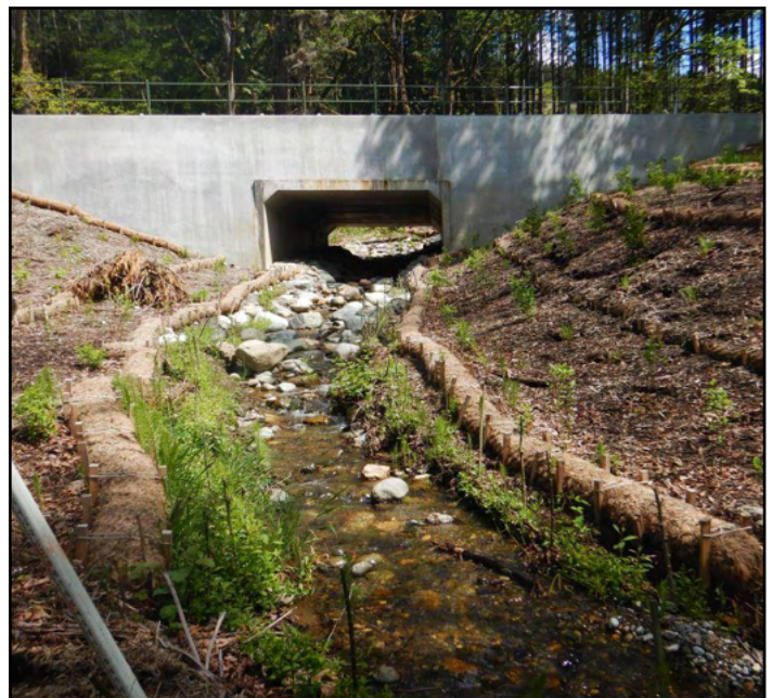
Figure 15. The new crossing is an 18 ft span by 14 ft rise 3-sided bottomless concrete culvert. This type and size of structure provides natural light penetration and allows the creek to naturally regrade if needed.
