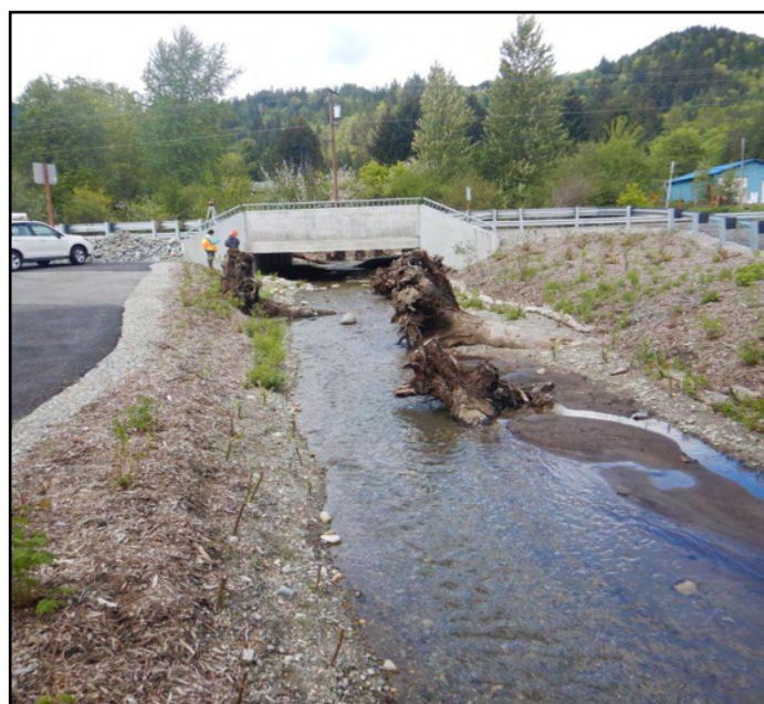
Figure 11. The new crossing is a 44 ft long, 20 ft span by 10.5 ft rise culvert. Adult salmon were observed in the culvert during a high flow event following construction.
