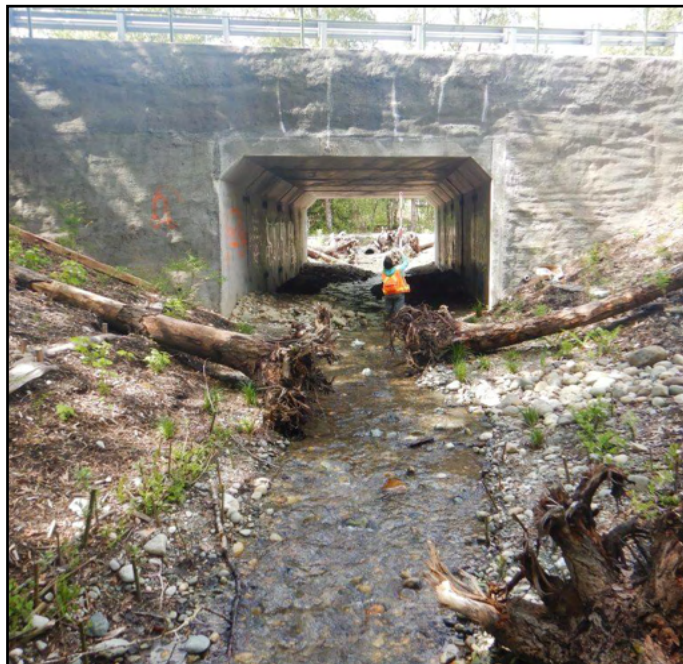
Figure 13. The new crossing is a 46 ft long, 16 ft span by 14 ft rise 3-sided bottomless concrete culvert. The 11 ft clearance height above the streambed allows natural light to penetrate through the structure.
