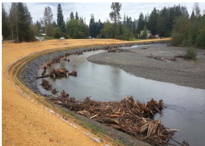
WSDOT crews stabilized the Pilchuck River banks and added woody material to the stream, resulting in increased habitat for aquatic species and protection of SR 92 from erosion.
