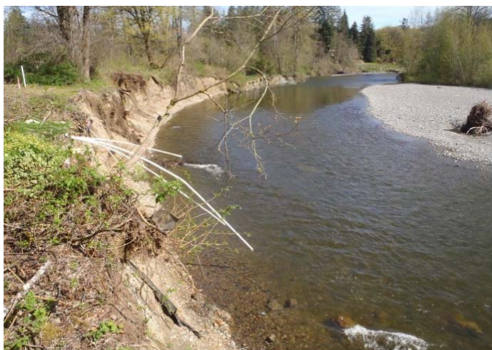
WSDOT crews stabilized the Pilchuck River banks and added woody material to the stream, resulting in increased habitat for aquatic species and protection of SR 92 from erosion.
