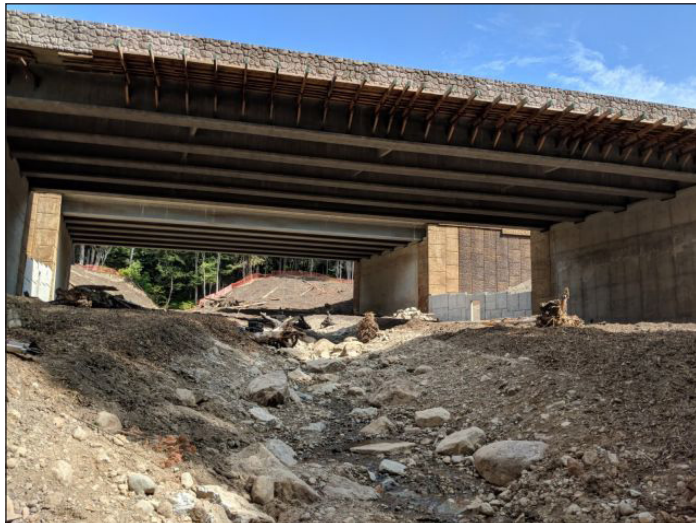
Figure 29. The new crossings are twin 120 ft (36.6 m) bridges for eastbound and westbound lanes of I-90. The new structures were installed as part of a larger transportation project on I-90 that added lanes and installed wildlife crossings between Keechelus Dam and the Stampede Pass interchange. The bridges allow unimpeded passage for fish and a variety of wildlife species through the Price Creek corridor and open over 1 mi (1.6 km) of habitat upstream for steelhead, resident trout, and bull trout.
