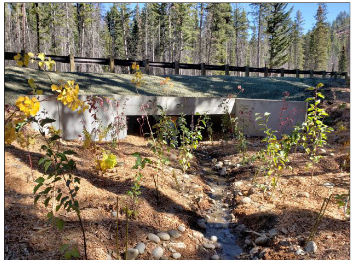
Figure 35. The new crossing is a 13 ft (4 m) wide by 7.5 ft (2.3 m) high concrete box culvert that restores access to 0.43 mi (0.7 km) of upstream habitat for steelhead and trout and facilitates use by small terrestrial wildlife.
