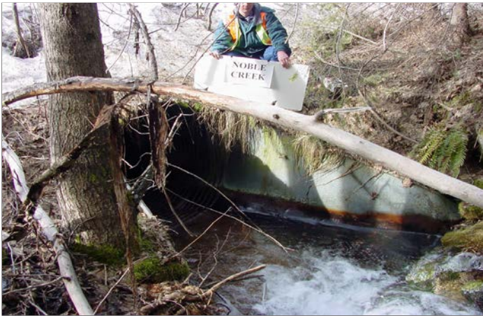
Figure 30. The old crossing was a 4 ft (1.2 m) diameter culvert. Noble Creek was previously classified as non-fish-bearing and passability was not assessed. Noble Creek was rerouted during the project and now meets physical criteria to be considered a fish-bearing stream.
