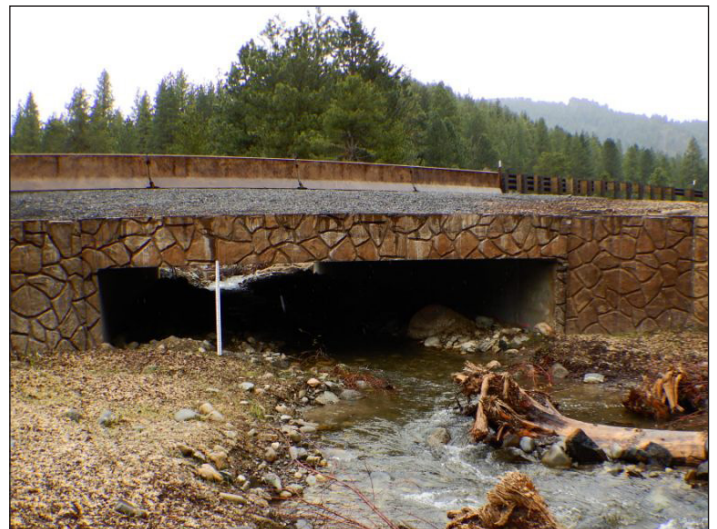
Figure 33. The new Mill crossing is a 75 ft (22.9 m) long by 25 ft (7.6 m) wide by 10.3 ft (3.1 m) high concrete box culvert that allows unimpeded fish passage for steelhead, resident trout, and bull trout. The project included installation of large wood and constructed stream meanders.
