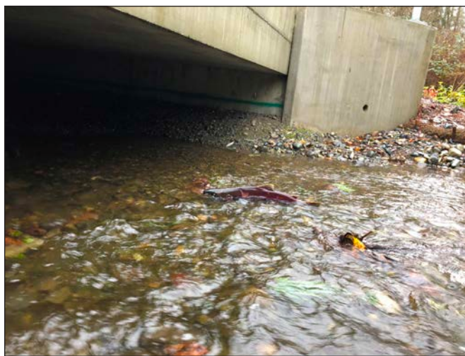
Adult coho returning to Green Creek through a new stream-simulation culvert constructed in 2017 on SR 900 in King County. (Zach Moore and Panos Stratis, WDFW)
