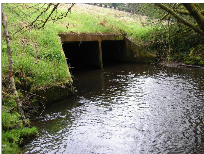
Figure 20. The old crossing was a double-box culvert 10 ft (3.0 m) wide by 8 ft (2.4 m) high on each side and was a fish passage barrier due to excessive velocity during high flow conditions.
