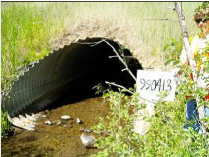
Figure 32. The old crossing, termed the Mill crossing, was a 9 ft (2.7 m) wide by 6 ft (1.8 m) high multi plate corrugated metal culvert installed in 1952. The crossing was a barrier to fish passage due to excessive slope.
