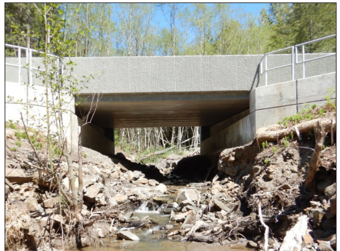
Figure 25. The new crossing is a 20 ft (6.1 m) wide concrete bottomless arch with secant pile walls that will allow the channel to vertically regrade over time. This correction provides access to 1.76 mi (2.8 km) of habitat upstream for coho, steelhead, searun cutthroat, and resident trout.
