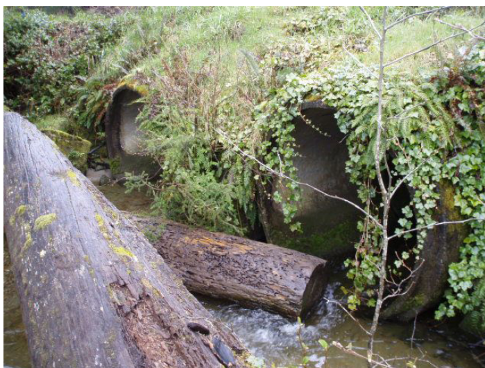
Figure 16. The old crossing consisted of two 6 ft (1.8 m) diameter concrete culverts. The majority of flow during low flow periods was conveyed through the left bank culvert. The crossing was considered a fish passage barrier due to excessive velocity through the structures during high flow conditions and a minimum depth barrier due to too little water during low flow conditions.
