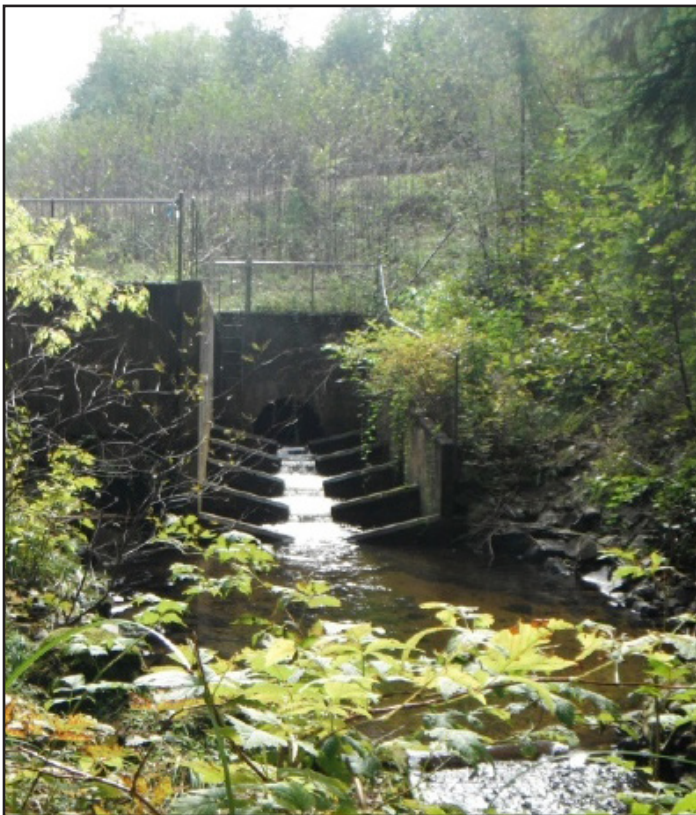
Figure 38. An example of a durable and efficient fishway on SR 401 at milepost 8.8 for Cement Creek.
