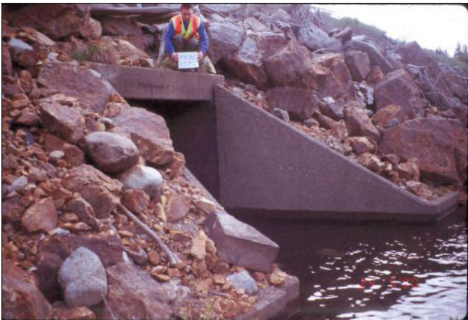
Figure 26. The old crossing was a 6 ft (1.8 m) by 6 ft (1.8 m) concrete box culvert that was a barrier to fish passage.
