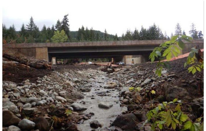
Figure 31. The new crossings are twin 120 ft (36.6 m) bridges for eastbound and westbound lanes of I-90. The structures were installed as part of a larger transportation project on I-90 that added lanes and installed wildlife crossings between Keechelus Dam and the Stampede Pass interchange. The bridges allow unimpeded passage for steelhead, trout, and a variety of wildlife species through the Noble Creek corridor.
