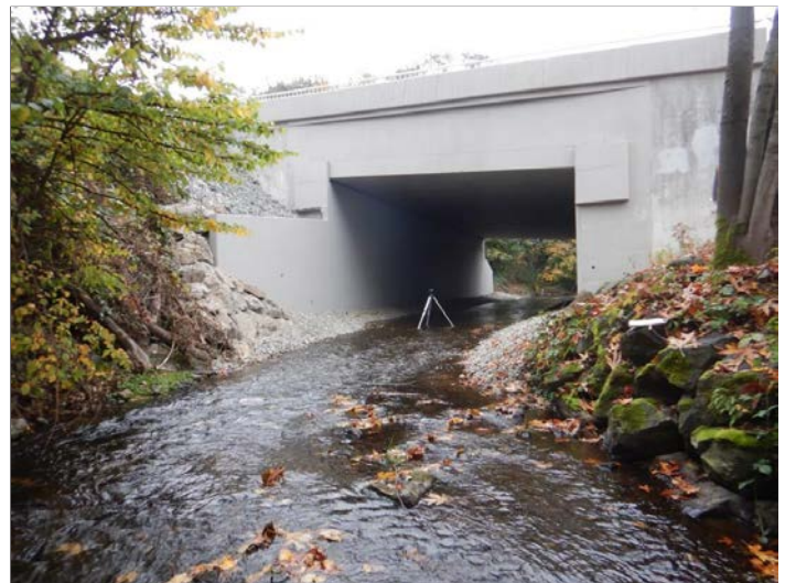
Figure 13. The new crossing is a concrete bottomless arch measuring 30 ft (9.1 m) wide by 23.5 ft (7.2 m) high that restores fish passage. The downstream grade controls are slated to be removed as part of a future City of Woodinville stream restoration project, which will bring the channel into an equilibrium slope through the SR 202 crossing.
