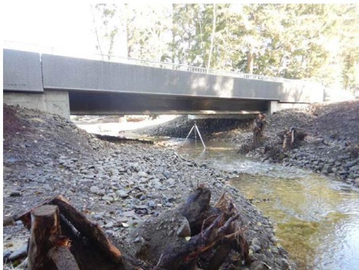
Figure 17. The new crossing is a full span concrete bridge with a 45 ft (13.7 m) opening that provides access to 3.6 mi (5.8 km) of potential habitat for fish. The project included installation of large wood upstream and downstream of the new crossing to provide bank protection and refuge from predators during high tide.
