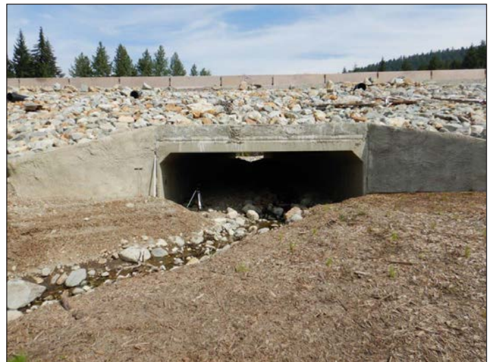
Figure 27. The new crossing was installed as part of a larger transportation project on I-90 that added lanes and installed wildlife crossings between Keechelus Dam and the Stampede Pass interchange. The new culvert is a stream simulation 25 ft (7.6 m) wide by 14 ft (4.3 m) high concrete box culvert that allows for unimpeded passage for resident rainbow, cutthroat, and bull trout.
