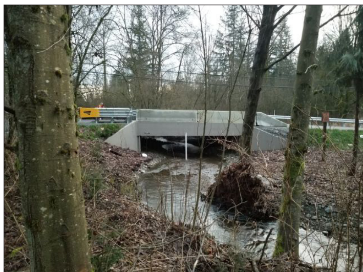
Figure 15. The new crossing is a concrete box culvert 19 ft (5.8 m) wide by 9.3 ft (2.8 m) high that allows unimpeded passage of fish and large wood through the structure. The project included installation of four pieces of wood at the outlet and a slight realignment to remove a sharp bend at the inlet. Two rock barbs were added inside the culvert to provide habitat complexity. Salmonids and a redd were observed upstream of the new culvert during the compliance inspection.
