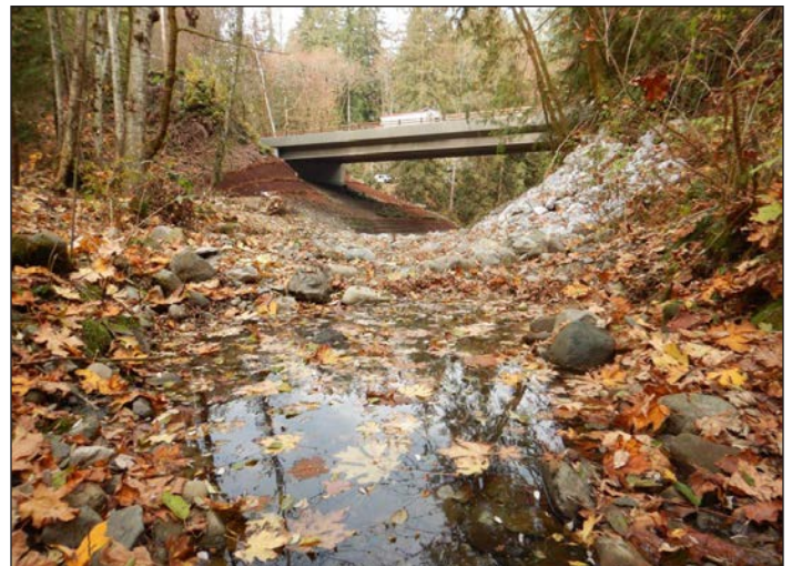
Figure 5. The new 127 ft (38.7 m) span bridge provides unimpeded access for salmon, steelhead, and trout to upstream habitat. The bridge reconnects the stream corridor and allows downstream movement of boulders and large wood in this seasonally high energy drainage.
