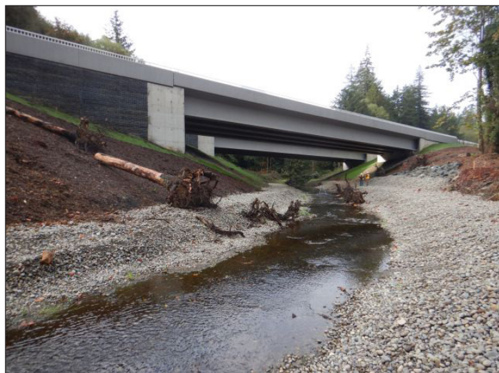
Figure 21. The new crossings are two 160 ft (48.8 m) long bridges for eastbound and westbound lanes. Large wood provides refuge for fish and increases stream habitat complexity. Correction of this barrier opens 13.6 mi (21.9 km) of potential habitat upstream for chum, Chinook, coho, steelhead, searun cutthroat, and resident trout.
