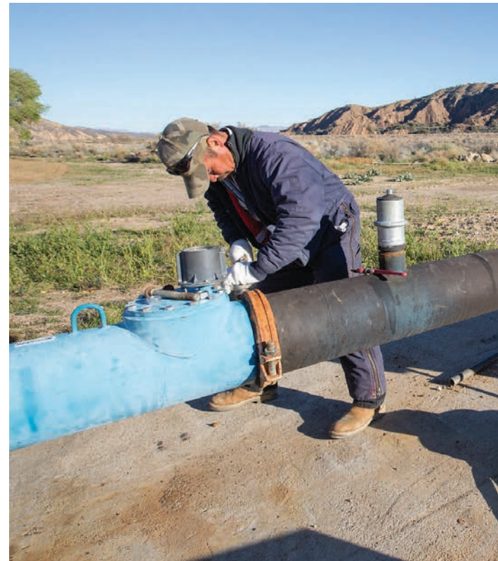
Marcel Emea repairs a seal on an irrigation pump. The orchards canal system.
