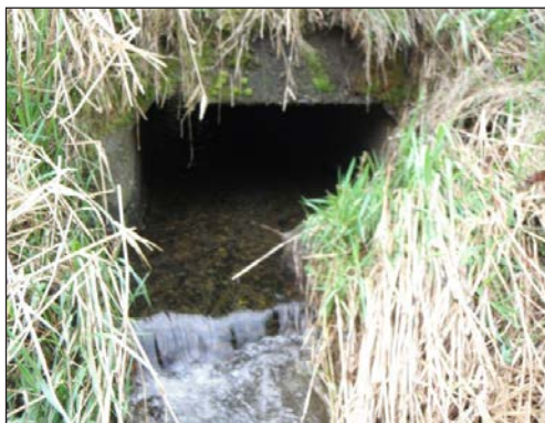
Figure 12. The old crossing on the west tributary (top) consisted of two culverts – a 4 ft (1.22 m) wide by 2.1 ft (0.65 m) high concrete box culvert plus a 1.5 ft (0.46 m) diameter round culvert. The site was considered a slope barrier. The old crossing for the east tributary (bottom) was an 8 ft (2.43 m) wide by 5.8 ft (1.78 m) high concrete box culvert that was a high flow velocity barrier.
