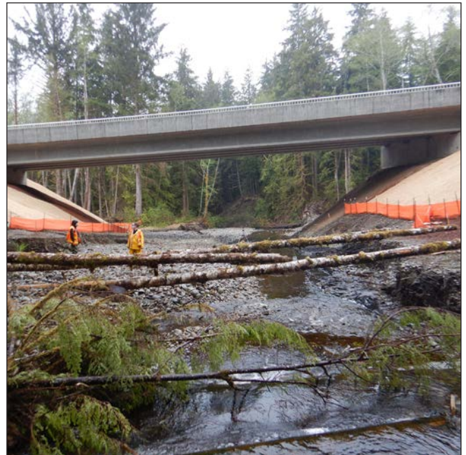
Figure 23. The new crossing is a 133 ft (40.5 m) span bridge that restores access to 9.56 mi (15.38 km) of previously blocked habitat for Chinook, coho, steelhead, and sea-run cutthroat.
