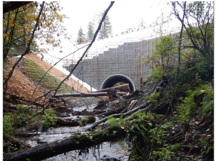
Figure 9. The new structure is a 26 ft (7.9 m) diameter structural plate steel culvert fitted with boulder cross-vanes to force the formation of step pools. Outside the structure, large wood and small slash were incorporated into the stream channel design. A deformable grade control, created with woody branches, helps to dissipate stream energy and reduces velocity entering the project reach.
