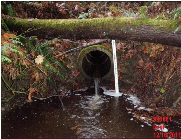
Figure 6. The old crossing was a 2 ft (0.61 m) diameter concrete culvert that was considered a total barrier due to an excessive hydraulic drop at the outlet.
