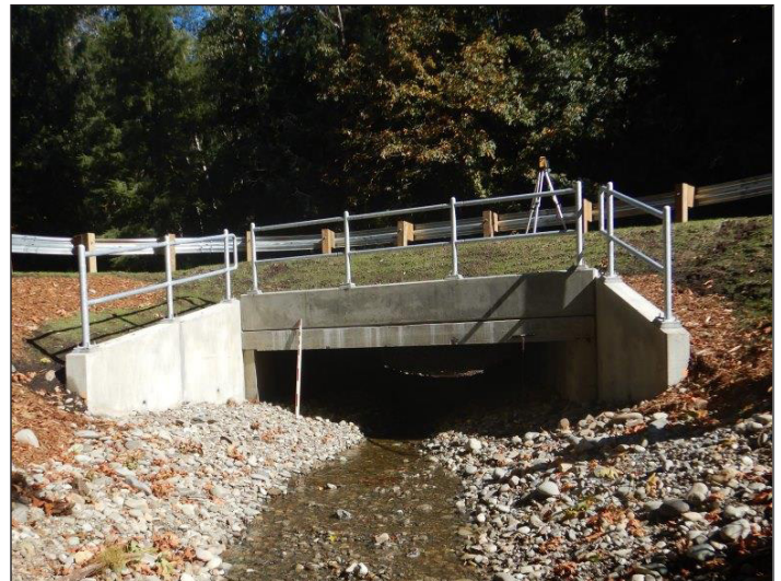
Figure 21. The new crossing is a 16.5 ft (5.04 m) wide by 9 ft (2.74 m) high concrete box culvert that allows unimpeded fish passage for coho, steelhead, sea-run cutthroat trout, and bull trout.
