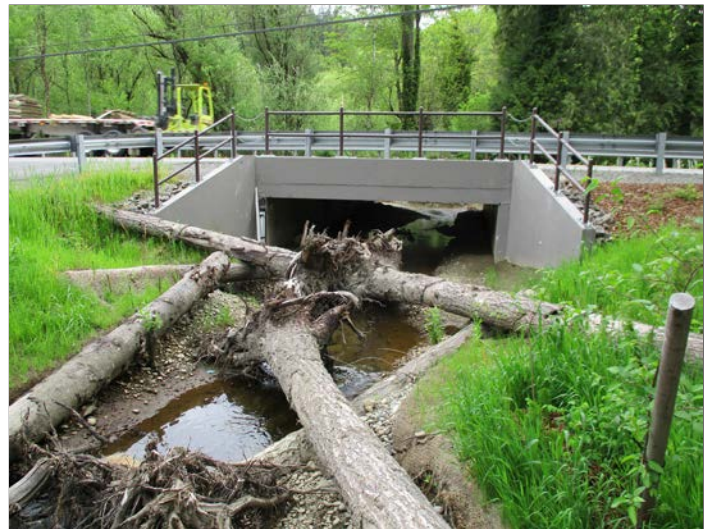
Figure 11. The new culvert is a 16.1 ft (4.9 m) wide by 9 ft (2.74 m) high concrete box culvert. Abundant large wood was placed both upstream and downstream of the new culvert to provide deep resting pools and refugia for fish.
