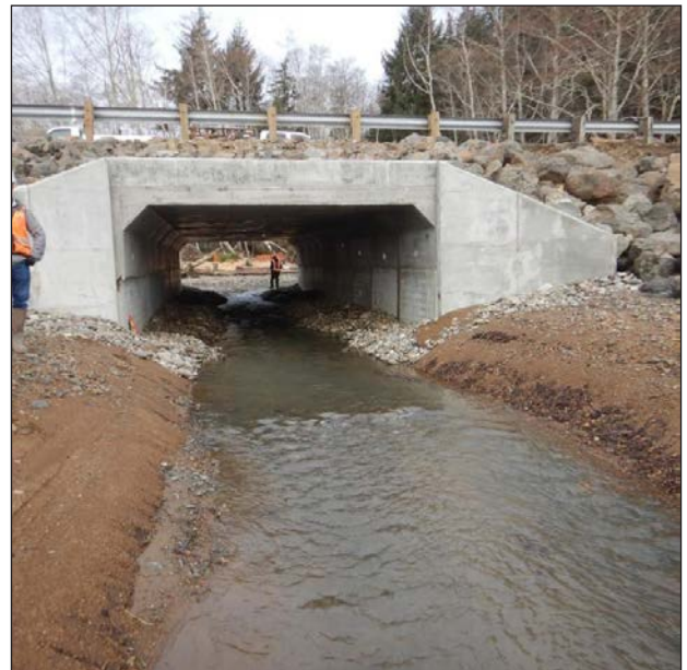
Figure 29. The new box culvert is adequately sized for the watershed and allows for fish passage in all tidal and flood events.
