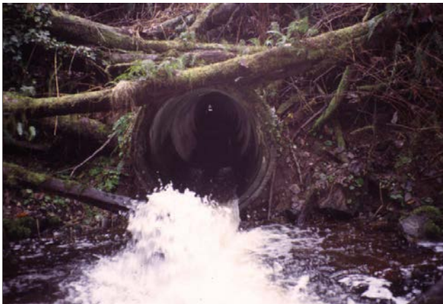
Figure 8. The old crossing was a 4 ft (1.22 m) round concrete culvert that was a barrier to fish passage due to an excessive water drop at the outlet, low water depth, and high velocity flow.
