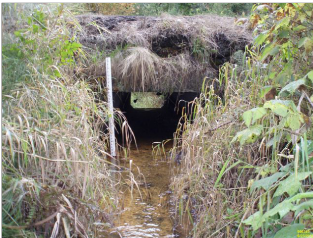
Figure 10. The old culvert was a 5 ft (1.53 m) wide by 3 ft (0.91 m) high concrete box culvert that was a high flow velocity barrier to migrating chum, coho, steelhead, and sea-run cutthroat trout.
