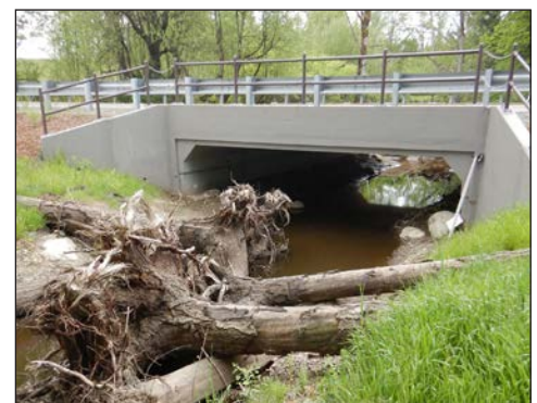
Figure 13. The new crossing for the west tributary (top) is a 12.3 ft (3.74 m) wide by 8.3 ft (2.54 m) high concrete box culvert. The new crossing for the east tributary (bottom) is a 23.1 ft (7.05 m) high by 10.5 ft (3.2 m) wide concrete box culvert. Both new structures provide unimpeded fish passage for adults and juvenile salmonids. Adult coho were observed transiting the new structures immediately following construction.
