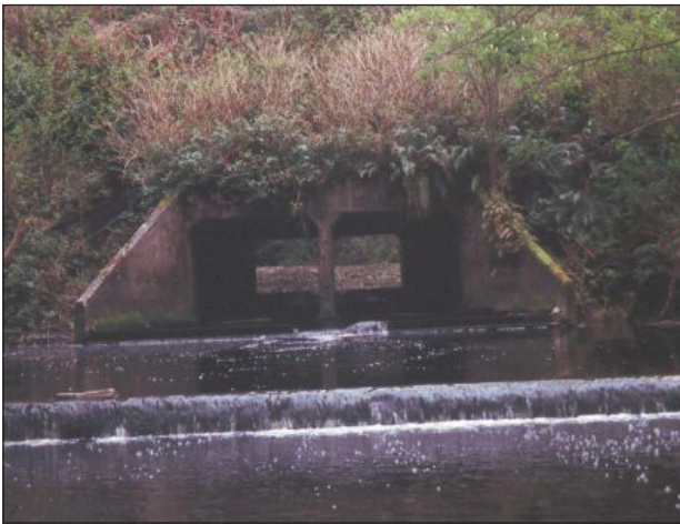
Figure 22. The old crossing was a twin box culvert with each opening measuring 8 ft (2.44 m) wide by 4 ft (1.22 m) high and retrofitted with 22 steel baffles and four log bed controls to aid in fish passage. Deteriorating baffles and an excessive water surface drop over the log controls caused this fishway to be assessed as a partial barrier.
