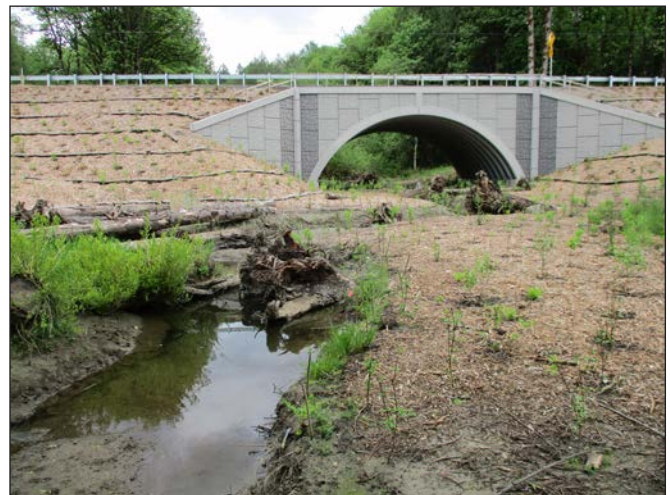
Figure 15. The new crossing is a 49.2 ft (15 m) span arch bridge. The innovative bridge design consists of fiberglass reinforced plastic sheet pile bolted to tubes that are filled with concrete. The structure is set on buried concrete footings. This modular design allows for quicker installation than a traditional bridge while providing high structural strength and light weight.
