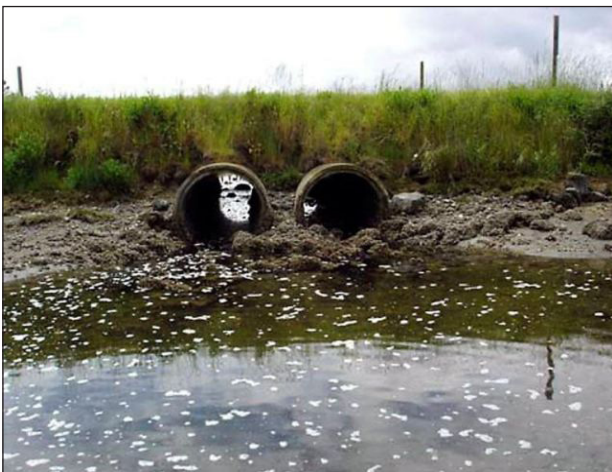
Figure 18. The old crossing on SR 116 consisted of two 5 ft (1.52 m) diameter concrete culverts that prevented adequate tidal exchange and was considered a partial barrier for fish passage.
