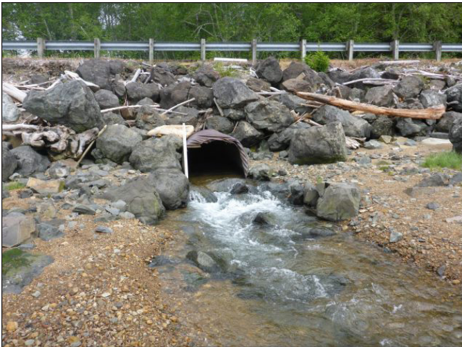
Figure 26. The old crossing was a 5 ft (1.52 m) diameter corrugated metal culvert that blocked Chinook, coho, steelhead, and sea-run cutthroat trout.
