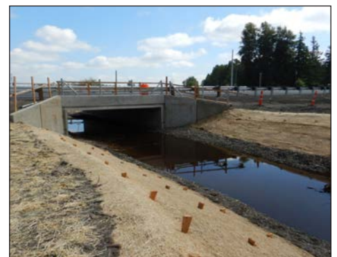
Figure 5. The lengthy I-5 culvert was replaced with three shorter structures. Two new structures were installed under the northbound (top) and southbound (bottom) lanes of I-5 and one under Zell Road. Both new structures are 18 ft (5.5 m) wide by 9.1 ft (2.78 m) high concrete box culverts. The new crossing on SR 548 is a 12.1 ft (3.69 m) wide by 6.2 ft (1.9 m) high concrete box culvert.
