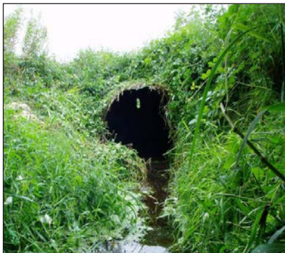
Figure 4. The old crossing on I-5 (photo) was a 5.5 ft (1.67 m) diameter corrugated steel culvert that was a high flow velocity barrier to adult fish. The 340 ft (103.6 m) long culvert extended under all lanes of I-5 and Zell Road. The old crossing on SR 548 was a 3 ft (0.91 m) diameter concrete culvert which was both a high flow velocity barrier and low flow depth barrier.
