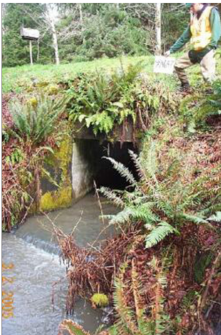
Figure 20. The old crossing was a concrete box culvert 5 ft (1.52 m) wide by 5 ft (1.52 m) high. The culvert was assessed as a high flow velocity barrier to fish passage.
