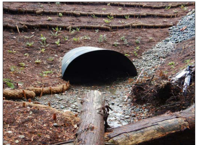
Figure 7. The new crossing is a 12 ft (3.66 m) diameter corrugated steel culvert coated in polymer to reduce corrosion. Additional consideration for small terrestrial species passage is reflected in the larger structure size. The project design included fish habitat complexity features by adding large wood in the channel both upstream and downstream of the new culvert.
