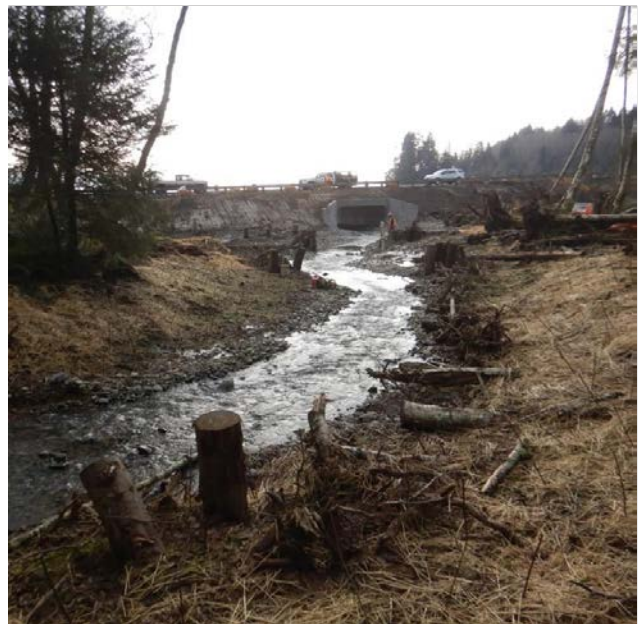
Figure 27. The new crossing is an 18.1 ft (5.52 m) wide by 12 ft (3.66 m) high concrete box culvert. The project includes restoration of approximately 175 ft (53.3 m) of stream channel upstream of the highway and enhancement of the floodplain to maximize connectivity at high tide. Juvenile salmon were observed utilizing pool habitat immediately after completion of the project.
