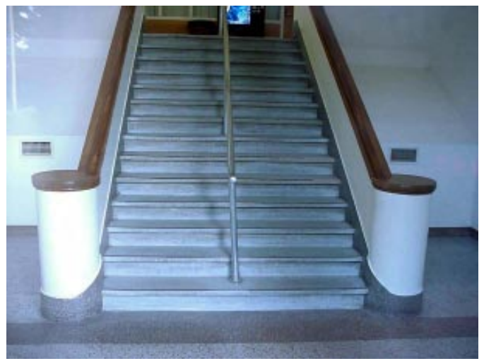
INTERIOR STAIR DETAIL.
