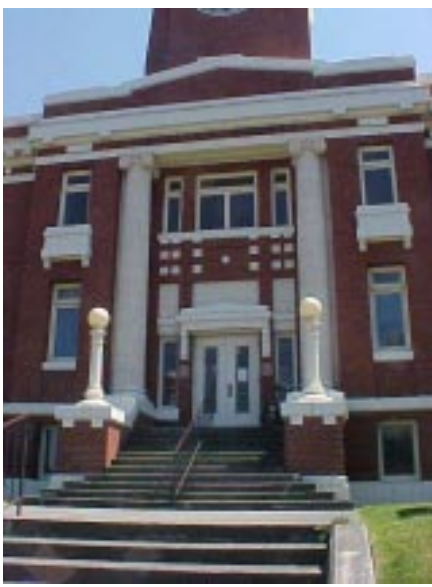
MAIN ENTRANCE DETAIL.
