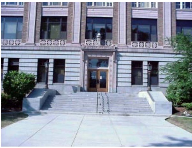
MAIN ENTRANCE DETAIL.
