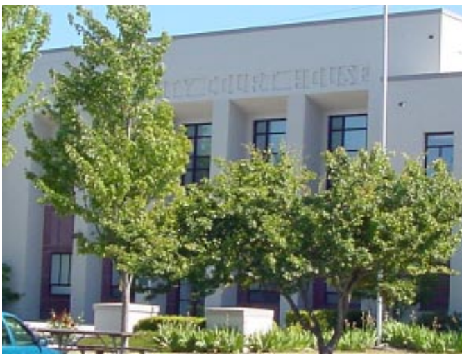
MAIN ENTRANCE DETAIL.
