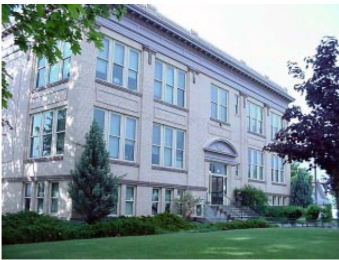
MAIN ENTRANCE DETAIL.
