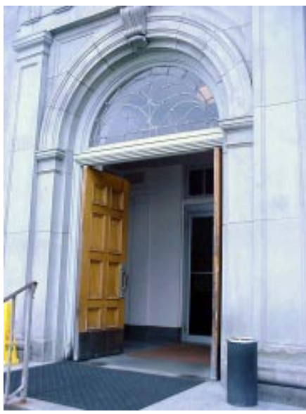
MAIN ENTRANCE DETAIL.
