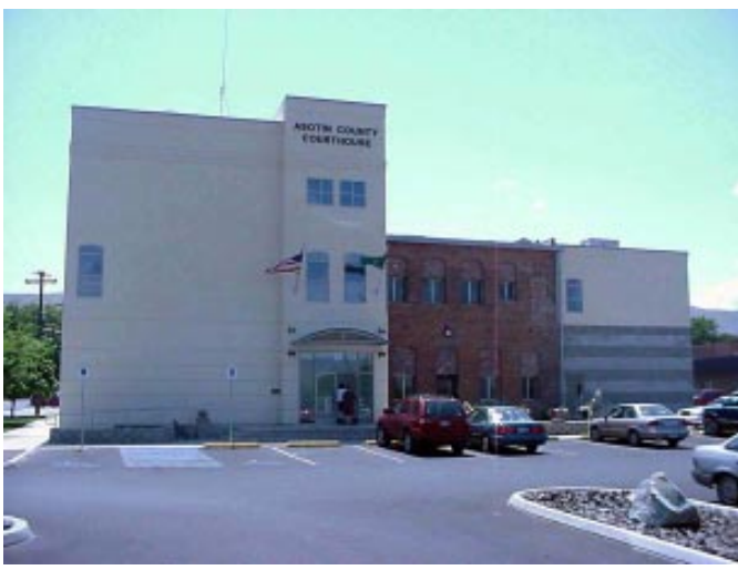
EXTERIOR NEW FACADE.
