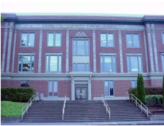
MAIN ENTRANCE DETAIL.
