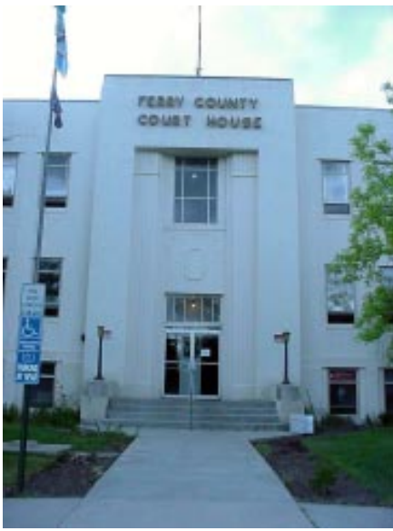
MAIN ENTRANCE DETAIL.
