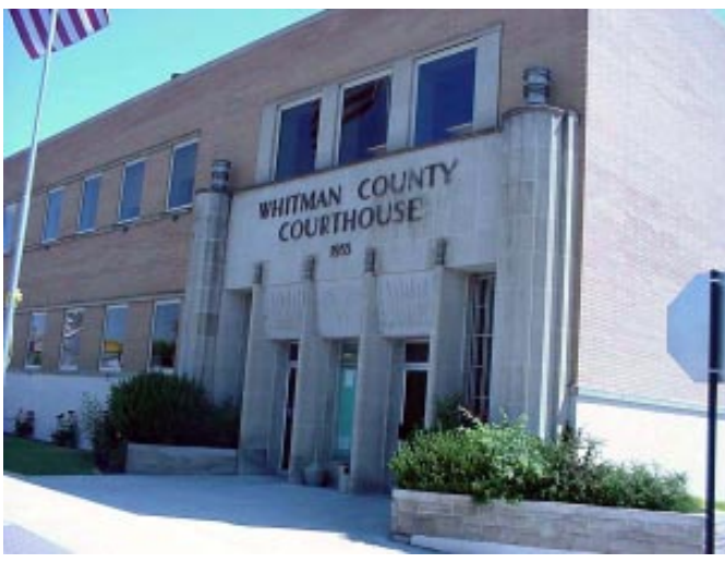
MAIN ENTRANCE DETAIL.
