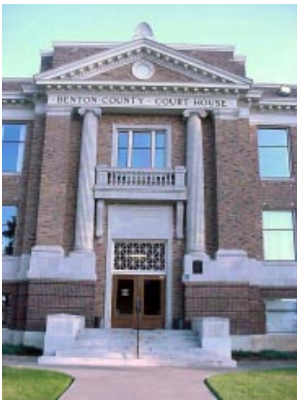
MAIN ENTRANCE DETAIL.
