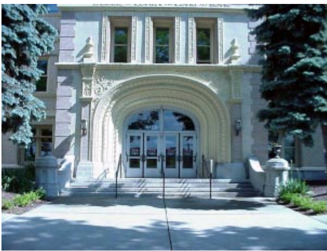
MAIN ENTRANCE DETAIL.
