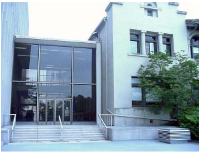
DETAIL OF CONNECTION BETWEEN HISTORIC AND NEW ADDITION.
