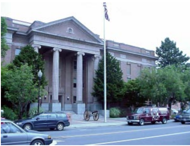
MAIN ENTRANCE DETAIL.
