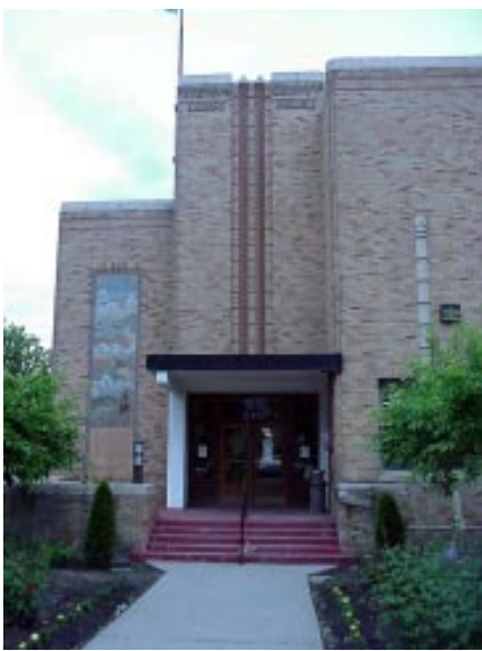
MAIN ENTRANCE DETAIL.
