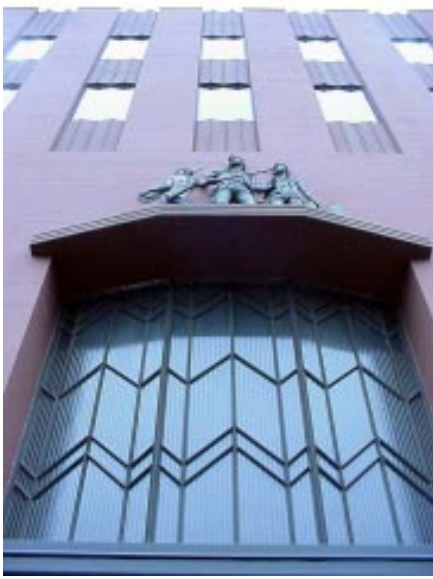
MAIN ENTRANCE DETAIL.
