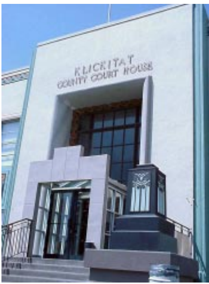
MAIN ENTRANCE DETAIL.
